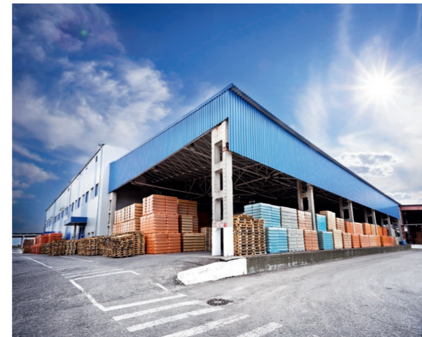
Outdoor fire detection close to buildings where almost no other detection technology is available with artificial intelligence based algorithms reducing unwanted alarms
